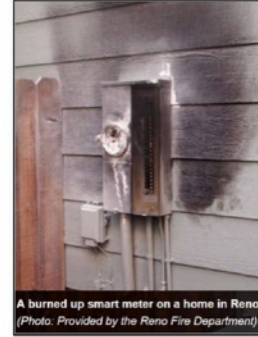
'smart' meter – burning, killing foliage
